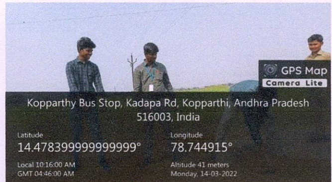
Laying of Road in Kopparthi Village, CK Dinne Mandal, Kadapa
